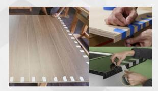
Apply masking tap on the edges & keep under pressure. Handling strength is received with in 2-3 hours, so finishing work can start. Full strength will be achieved with in 24 hours under room temperature.
