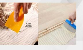
Stir the contents of the glue container just before application & spread the glue uniformly with a plastic notch spreader, first on the old laminate (scratch one) and then on fresh laminate (new one).
