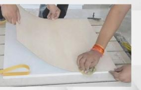
Once the tack is formed and the film turns transparent, paste the surfaces properly. Bring the laminate in contact to **HAMMER HI-BOND** coated ply surface and make proper alignment.
